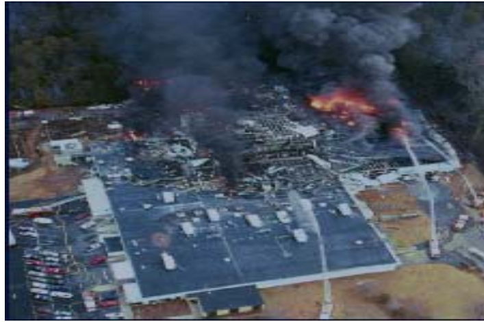
Picture showing Dust Explosion and Fire
